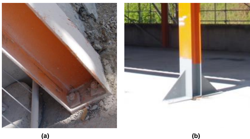
Figure 4 – Change in support conditions: (a) Fixed support - previous situation. (b) Clamping support - current situation .
