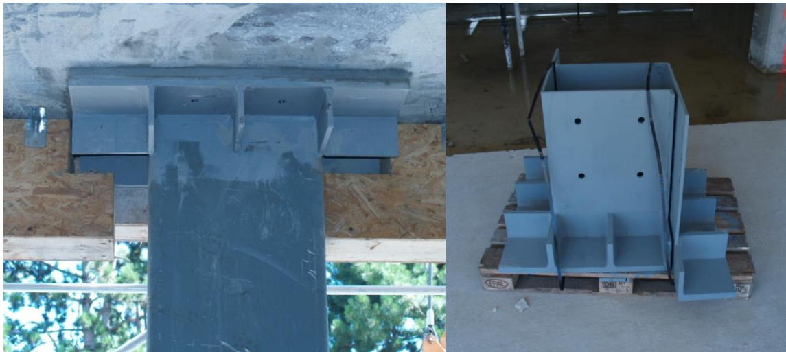
(a) (b) Figure 5 - (a) (b) Steel capitals in the heads of columns.
